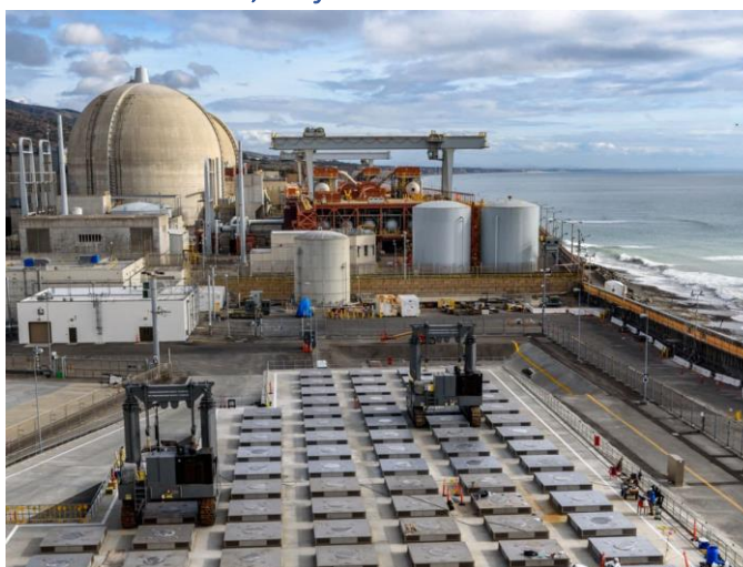
Figure 5-5. Square Tops of Spent Fuel Storage Silos at SONGS Visible in the Foreground
