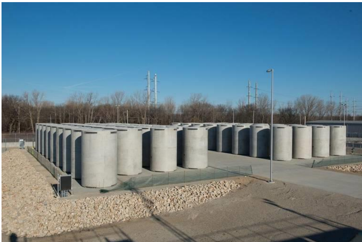
Figure 3-5. Spent nuclear fuel in dry cask storage at the Zion Nuclear Power Plant site.
