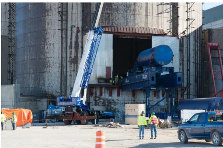
Figure 6-2. Large reactor components being removed during decommissioning of the Zion site
