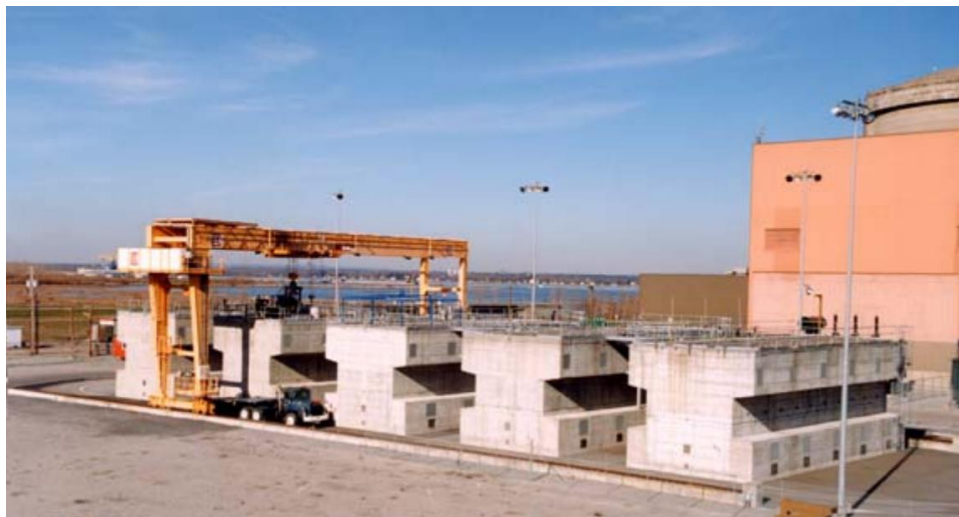
Figure 5-4. Large Modular Air-Cooled Storage (MACSTOR) units for spent fuel at Gentilly-2
