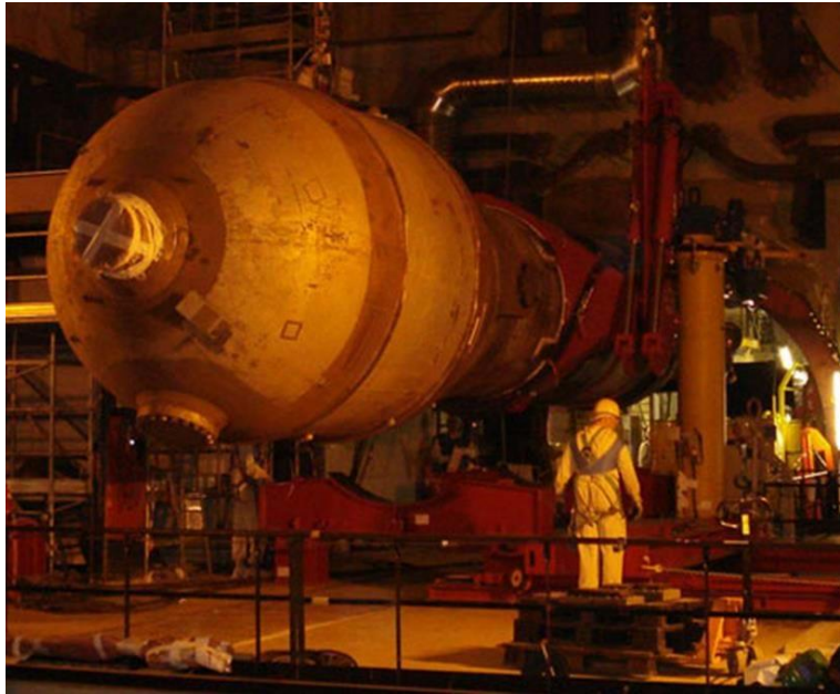
Figure 5-11. Removing the steam generator from the Chooz-A nuclear power plant.
