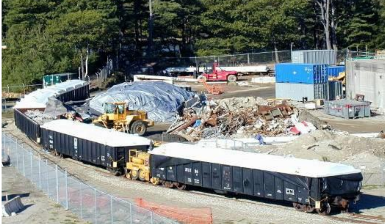
Figure 3-6. Bulk decommissioning waste being prepared for shipment at the Maine Yankee site.
