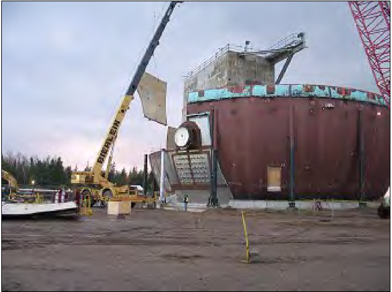
The Big Rock Point steel containment dome being dismantled.
