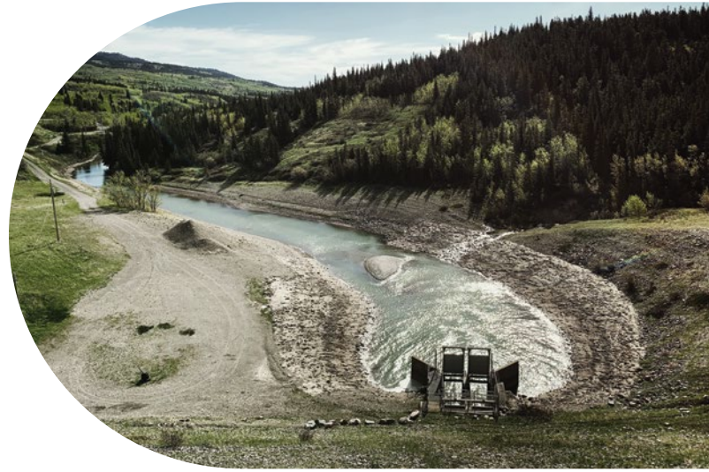
Figures 13: View of Lake Sherburne and spillway in Glacier National Park, Montana. Credit: Ethan Johnston.
