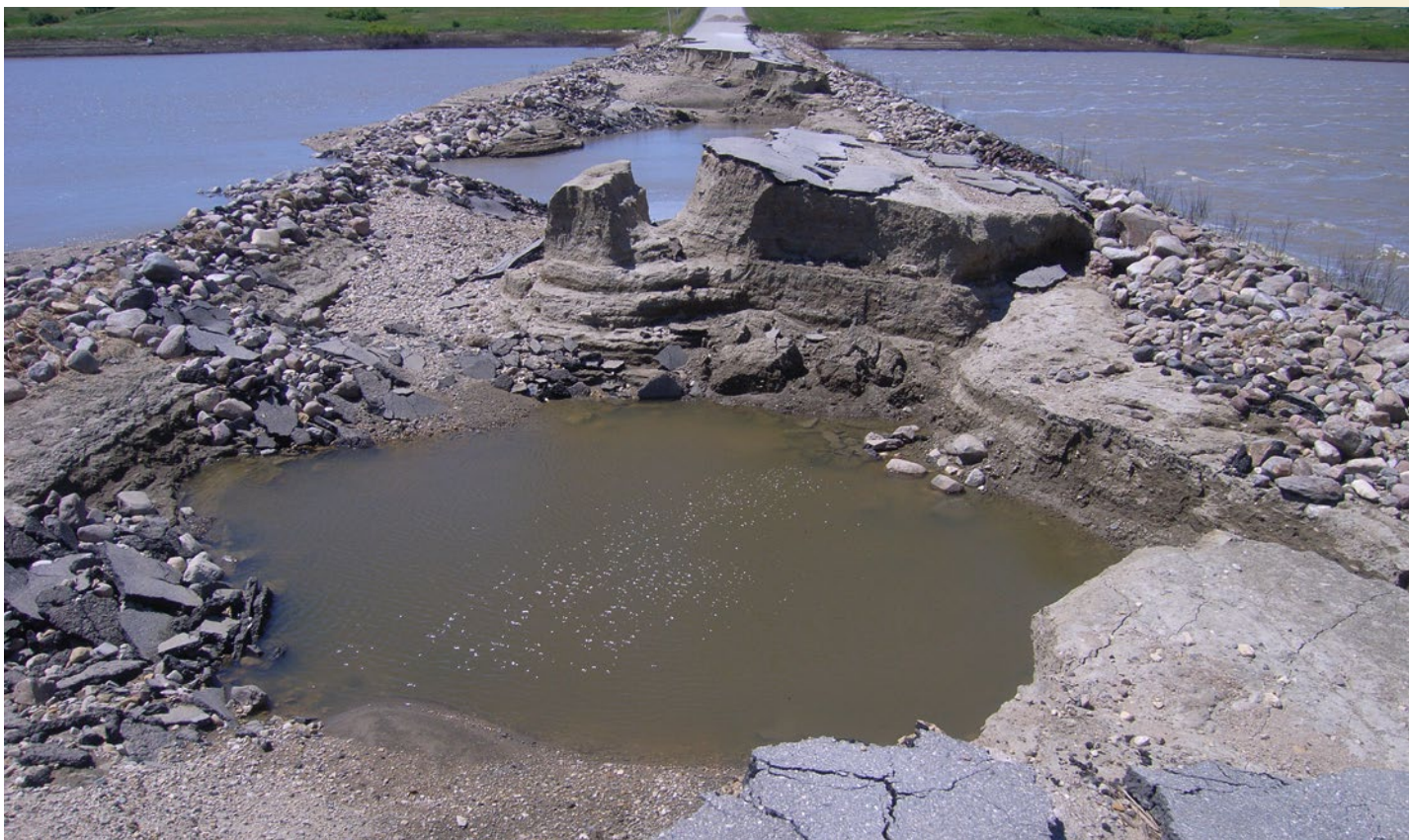
Image 15 Road washout caused by 2011 flood
