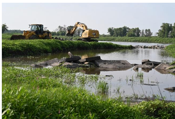
Drayton Dam Fish Passage construction. Image from USACE.
