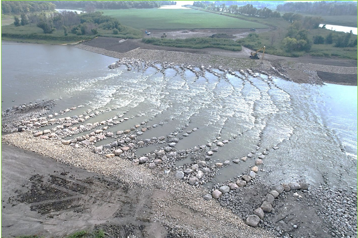
Fig. 4 – The newly constructed rock-arch-rapids at the former Drayton Dam site, ND.
