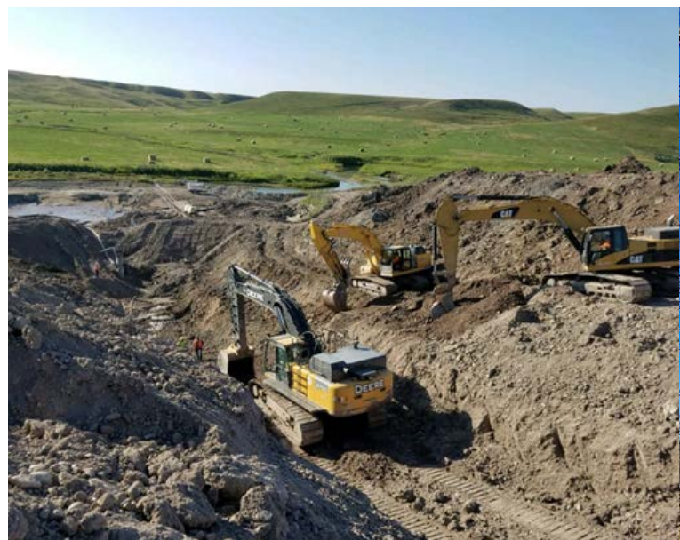
The Drop 5 stilling basin in the St. Mary Canal, used to reduce the velocity of the water, is being excavated and dewatered. Credit: John Kilpatrick
