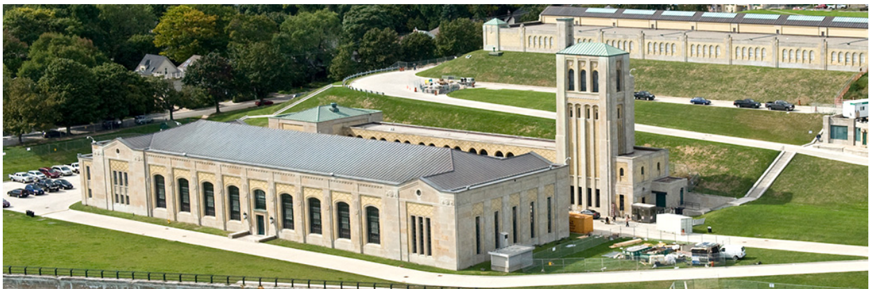
Figure 5-1: RC Harris Water Treatment Plant, Toronto, Ontario. Photo Credit: City of Toronto website: https://www.toronto.ca/services-payments/water-environment/tap-water-in-toronto/fast-facts-about-the-citys-water-treatment-plants/ .
