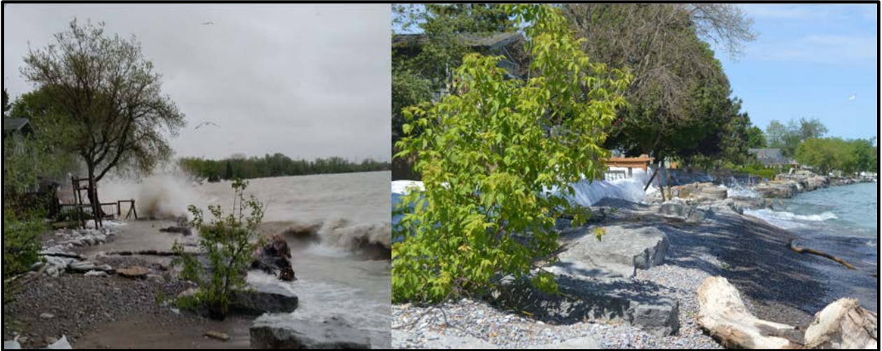
Figure 5-29: Cedar Crest Beach Road. The photo on the left was taken May 25, 2017. Photo credit: Clarington Fire and Emergency Services. The photo on the right was taken June 14, 2017. Photo credit: ECCC.
